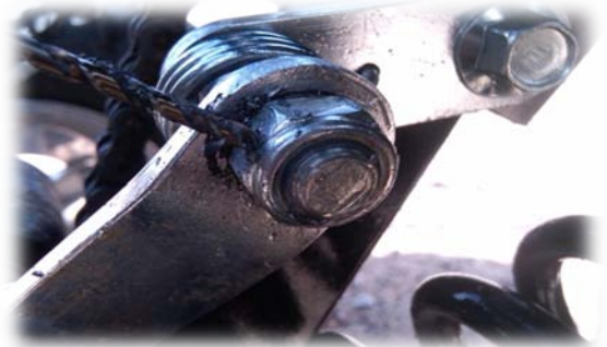
STEP 2: View of Drilling the Nut
